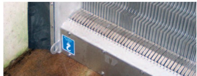
Example of a screen which is suitable for channel installation such that screenings are lifted at bottom level.
