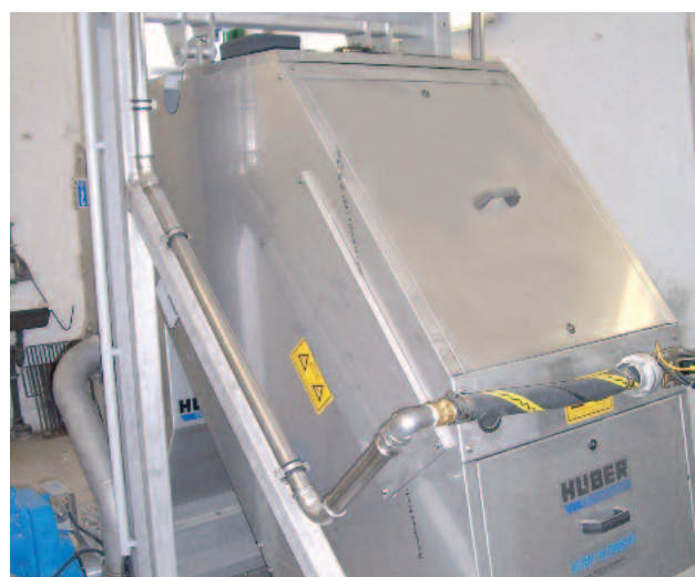
Fully enclosed, odour-free STEP SCREEN® Flexible SSF
