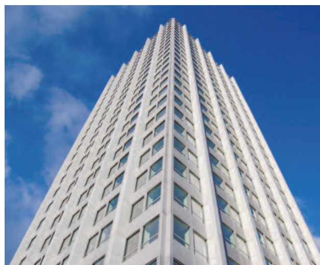
Climatisation of an office building with the HUBER ThermWin® system
