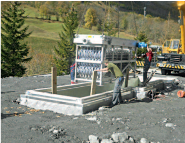
Wastewater from a swimming bath, about 450 kW heat output used to heat the swimming bath
