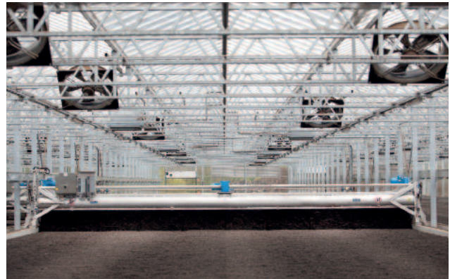
HUBER Sludge Turner SOLSTICE® for solar sewage sludge drying
