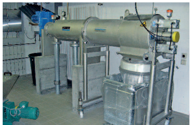
HUBER Sludgcleaner STRAINPRESS® – Continuous pressurised foreign material separation
