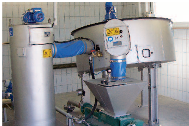
Unique sludge thickener: HUBER Disc Thickener S-DISC
