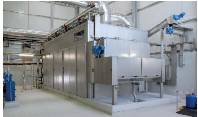
HUBER Belt Dryer BT for sewage sludge drying up to > 90% DS
