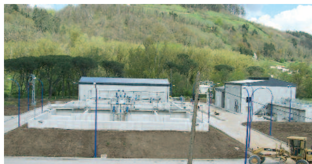
4 VRM® 30/448 units installed on the municipal WWTP Arenas de Iguna, Spain
