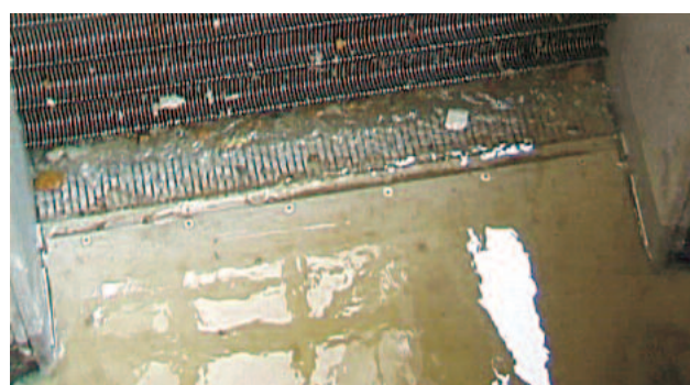
Example of a STEP SCREEN® Vertical SSV installed such that screenings are lifted at bottom level
