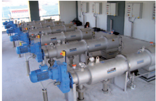
STRAINPRESS® – Continuous pressurised foreign material separation
